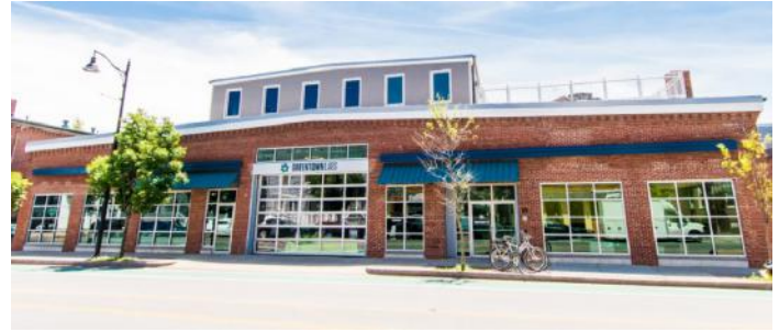
Photo: Greentown Labs
